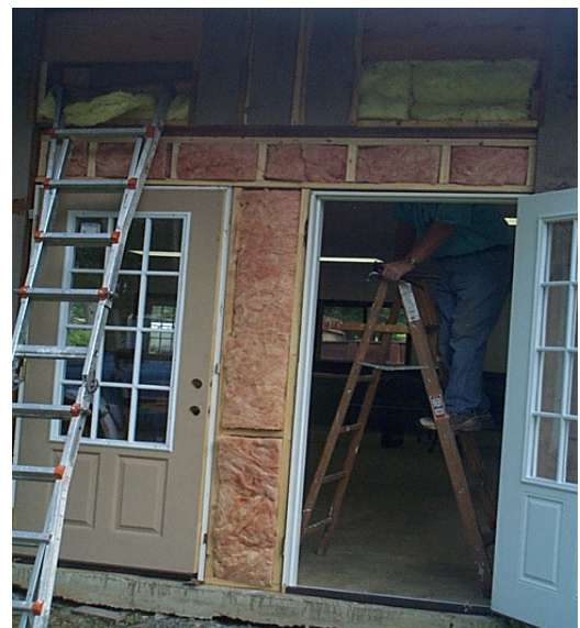
ONGOING WORK AT CAMP BADGER
